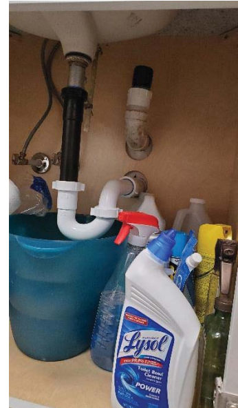
Vent re-installed vertically.
