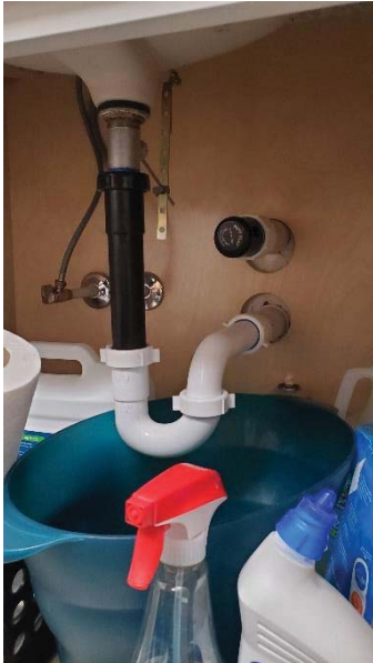
Vent installed horizontally.
