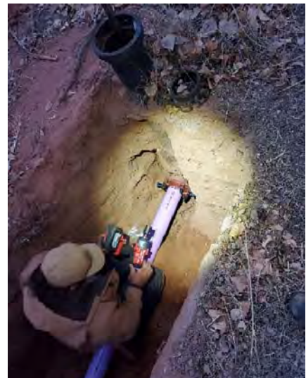
Mike is bolting in our irrigation line to the main valve by the irrigation well house.
