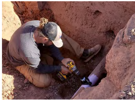
Mike installing a saddle on our 6" irrigation line.
