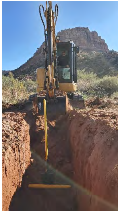
Ricky is trenching our irrigation line across Hildale Street over the gas line.
